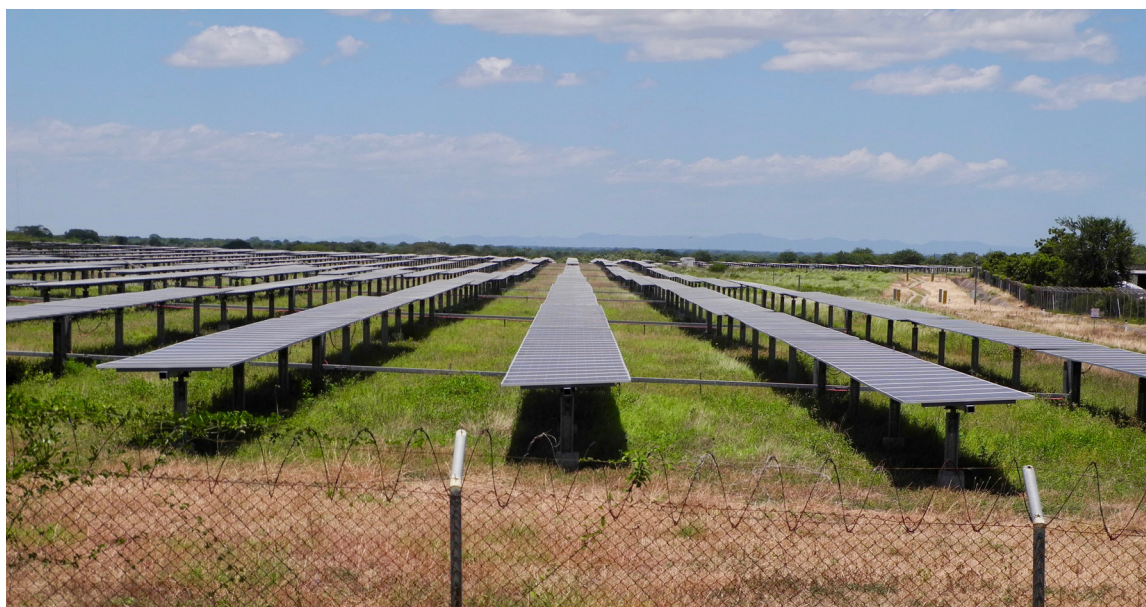
A solar park in Agua Fria, Nacaome, Honduras. Credit: Criterio.hn
